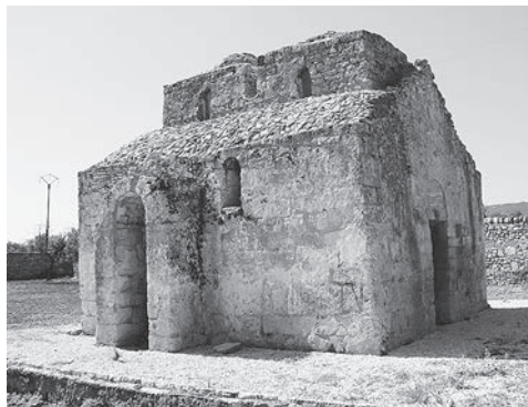
Il. 32. Seppanibale, church. Exterior view (photo: J.-P. Caillet)
