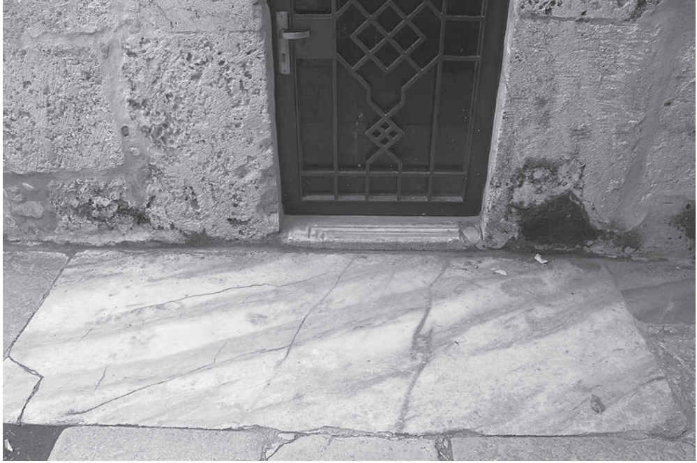
Il. 25. Marble chancel screen panel, reused as a threshold. Photo credit: A. Zelikman (2019)
