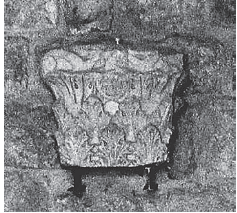
Il. 21. Late-Roman Corinthian capital, incorporated into the Late Islamic wall. Type 5 (mixed). Photo credit: S. Tarkhanova (2019)
