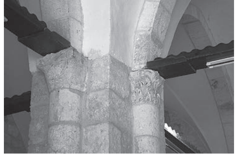
Il. 18. Roman Corinthian capitals reused in the Crusader church. Converted into the mosque. Photo credit: S. Tarkhanova (2019)
